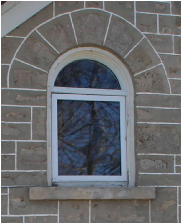
Figure 17 replaced upper window, 6581 Highway 6
