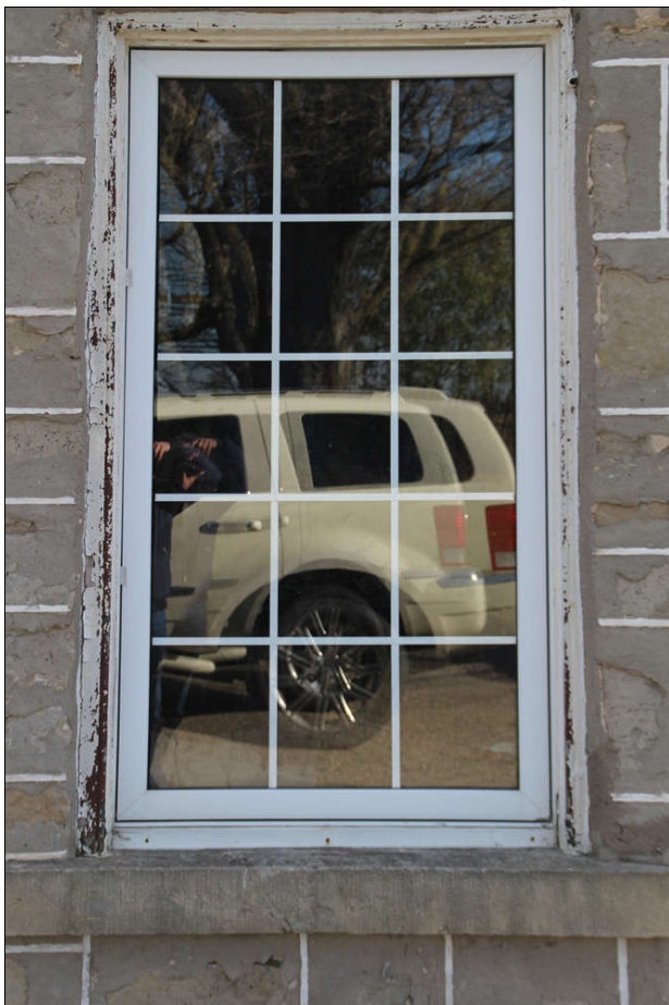
Figure 19 vinyl replacement window, 6581 Highway 6
