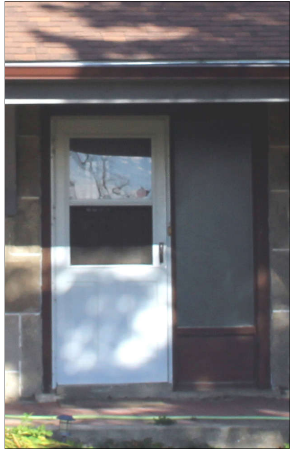
Figure 21 front door, 6581 Highway 6
