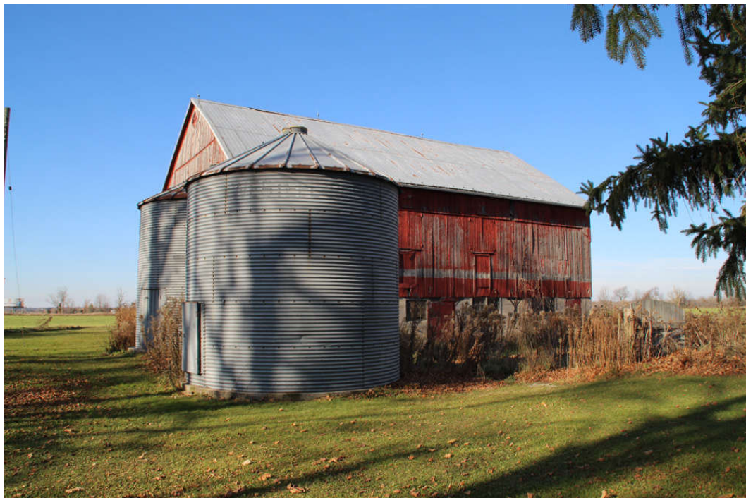
Figure 22 bank barn & storage bins, 6581 Highway 6
