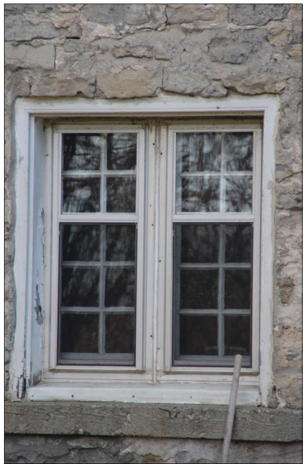
Figure 20 original 4/6 window, 6581 Highway 6
